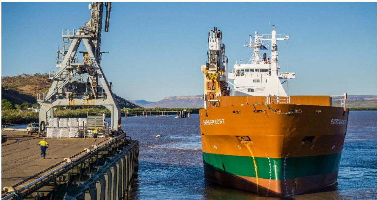
Figure 12: Vessel loading activities at Wyndham Port
